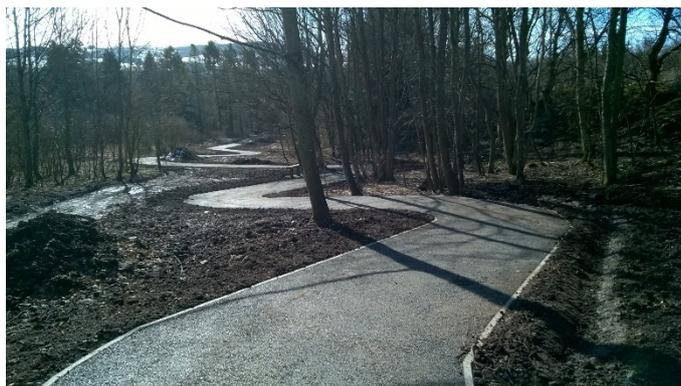
Two link paths running north into Auchterarder were widened, drained and given a sealed surface and the cemetery road was reconstructed with a whin dust surface treatment. To increase the utility of the path particularly in the winter months, solar powered stud lights were installed. Scottish designed units intended for Scottish light conditions were used to give the best results.
